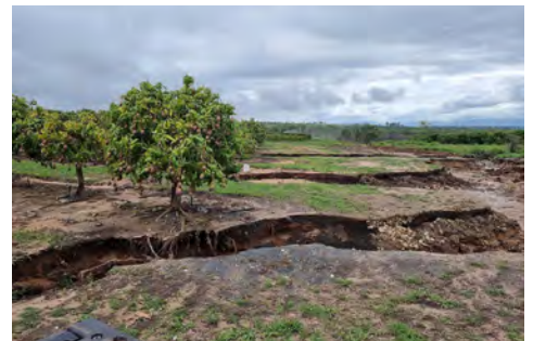
Washouts restricted access to some blocks
